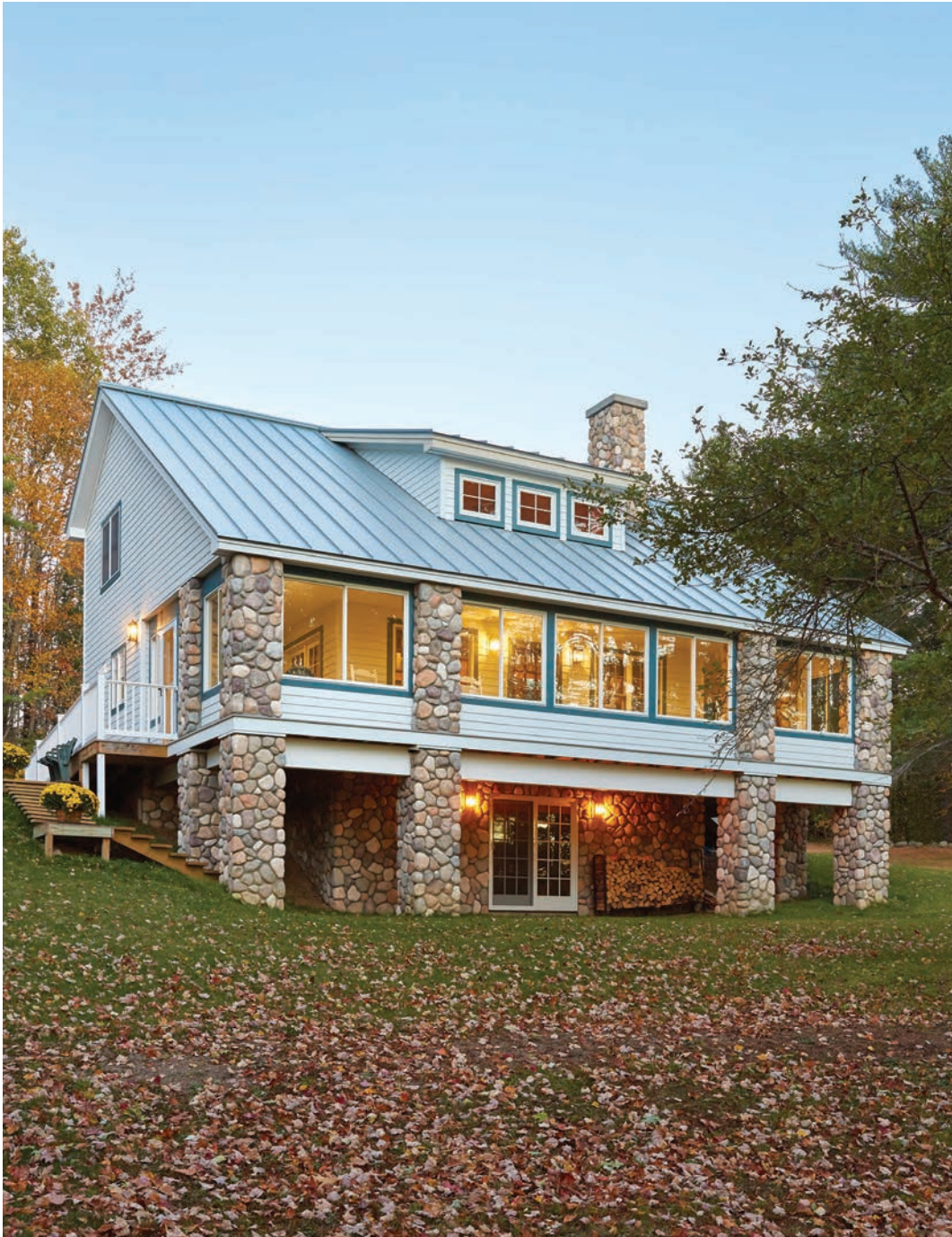
left An outdoor shot of the lake house provides a look at its Hardiplank exterior and fieldstone pillars and foundation. The glassed-in porch ensures that the tranquil lake view can be enjoyed in all weather.
